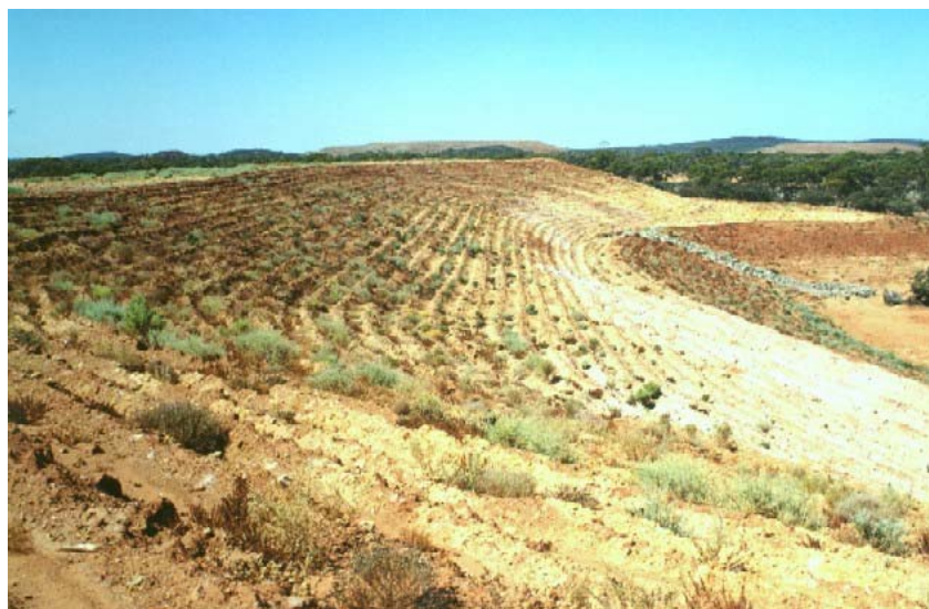
Figure 27. A batter slope that has been contour ripped to produce “bank and trough” physical resource regulating means. There are no signs of lateral flow in the troughs and hence no rills or gullies have formed.
