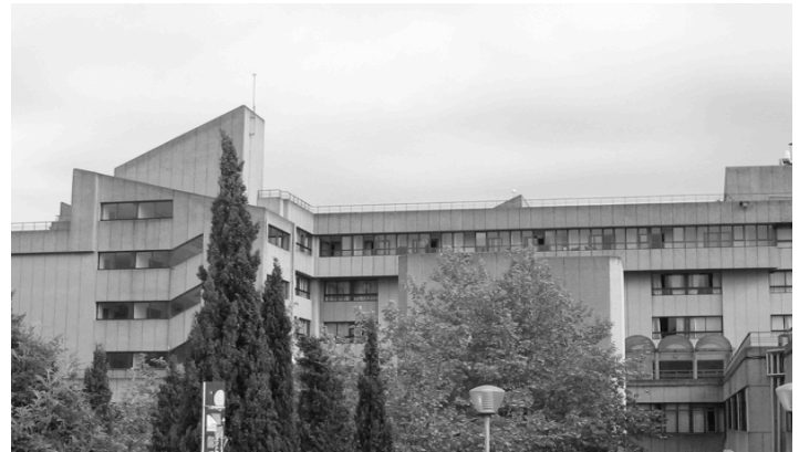
Figure 4. Monte da Condesa building in Santiago.
