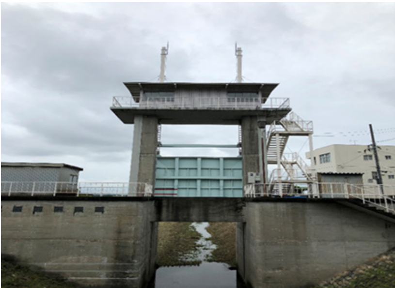
Figure 5 Flood control infrastructure in Gifu, Japan
